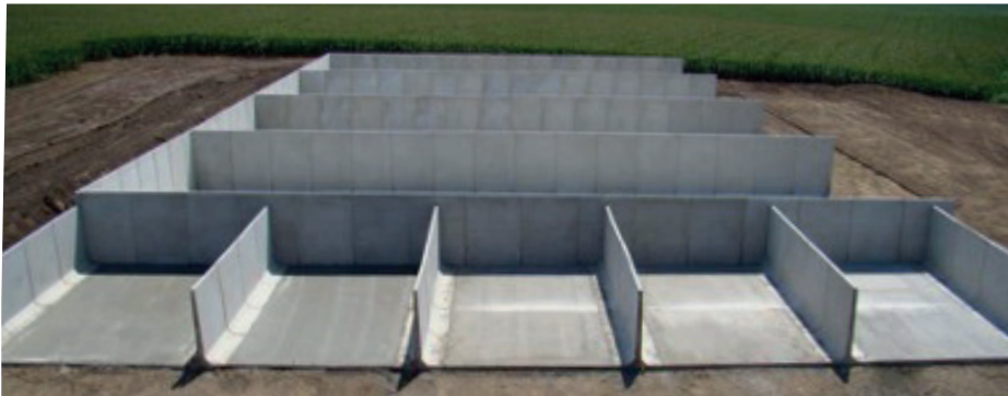
Figure 5 – Example of numerous large concrete paddocks (source: Hanson Silo)
