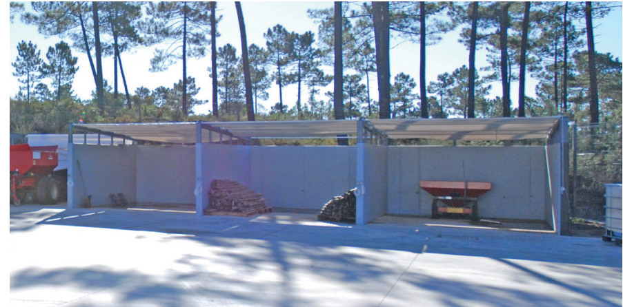
Figure 2. Example of storage bays
