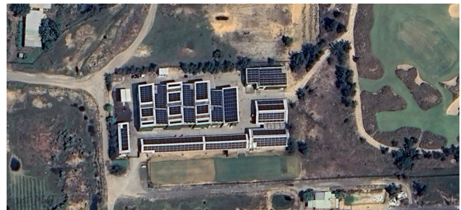
Figure 3. Solar Panel already installed but not being used
