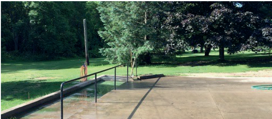
Figure 4. Simple sloped maintenance facility wash pad
