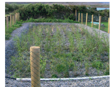
Figure 6. Simple constructed reed bed filter
